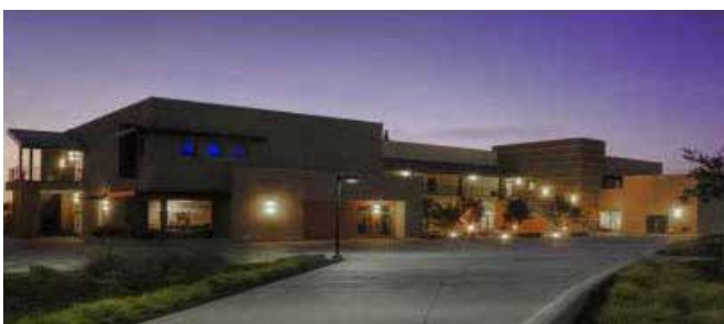
ALLIED SCIENCE & NURSING BUILDING* Allan Hancock College, Santa Maria Construction Cost: $18.8M
