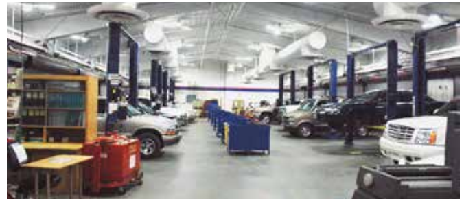
FRESNO CITY COLLEGE APPLIED TECHNOLOGY MODERNIZATION State Center Community College District, Fresno Construction Cost: $12M
