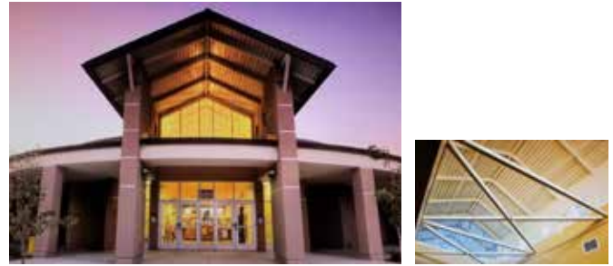
ALLAN HANCOCK COLLEGE SKILLS CENTER* Allan Hancock Jt. Community College District, Santa Maria Construction Cost: $9.2M
